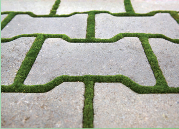
Permeable pavers reduce storm water runoff, thus less polluted water is likely to enter our waterways.
